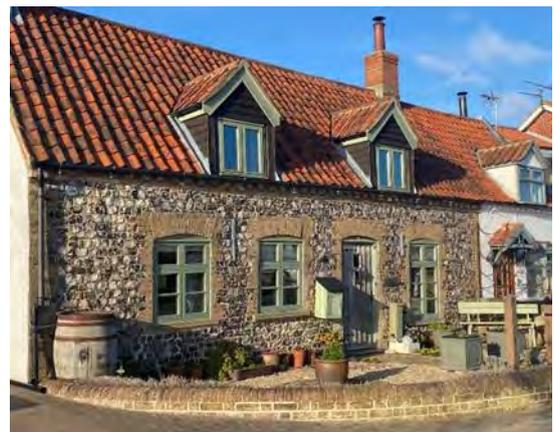
Above right: single storey flint cottage in Reedham with red pantile roof with dormer windows lighting accommodation in the roof space.
