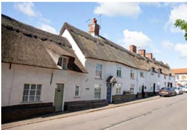
Above left: Thatched cottages in Ludham, with painted brick, render and timber joinery and building line directly on the pavement.
