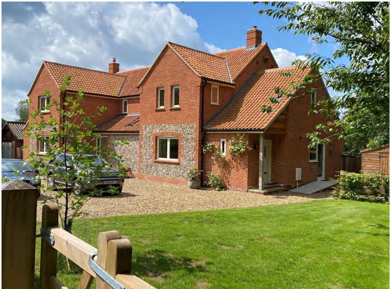
Above: a new home in Belaugh makes good use of traditional materials including timber joinery, red brick, flintwork and red clay pantiles. The massing of the building is successfully reduced by the projecting gables and varied roof forms.
