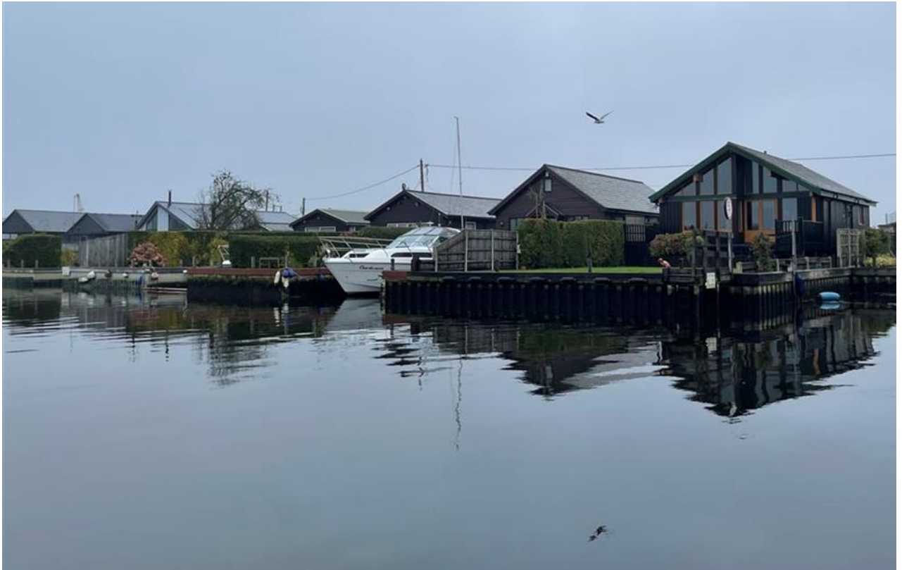
Above: Pitched roofs of varying pitches but consistency of orientation and no dormers on these 'shed-type' chalets at Brundall.
