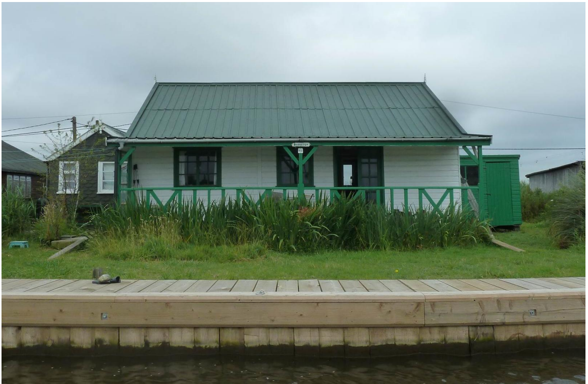
Above: A simple shed-type chalet positioned parallel to the river Thurne at Potter Heigham. The metal roof overhangs a verandah and the building has simple fenestration in a contrasting colour to the timber cladding. There is a decorative timber balustrade and finials on the roof.
