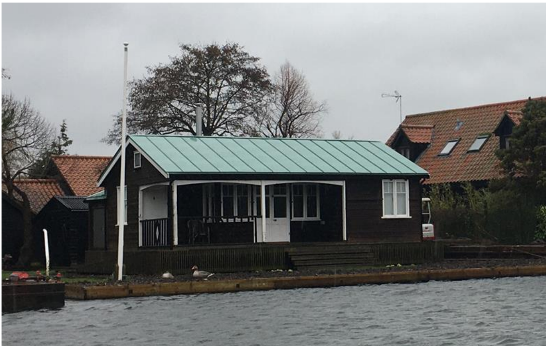
Above: Typical shed-like chalet on the river Bure at Horning. The building has a simple form and fenestration which is painted to contrast with the timber-clad walls, with a profiled metal roof and verandah.
