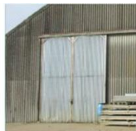
Metal sheet cladding
