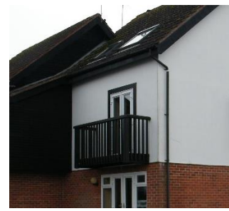
Mix of cladding materials
