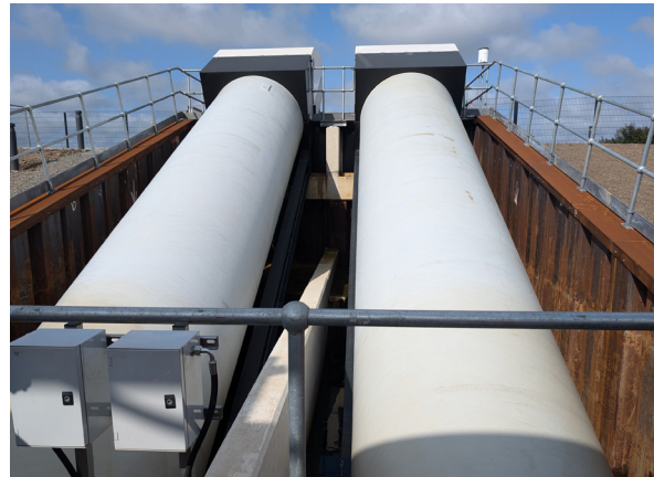
A new drainage pump at Norton's on the Yare helps manage both flood protection and water retention, supporting the carbon-rich floodplain and nature conservation. Andrea Kelly
