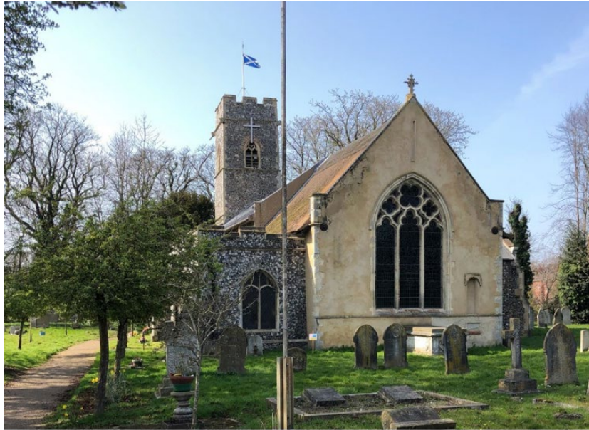
Figure 23- St Andrews Church
