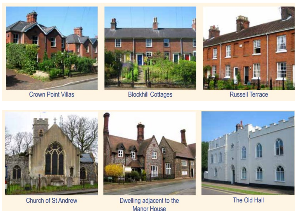
Figure 24- Pictures of properties in the TNCA Source: Trowse with Newton Conservation Area Character Appraisal and Management Plan (2012)
