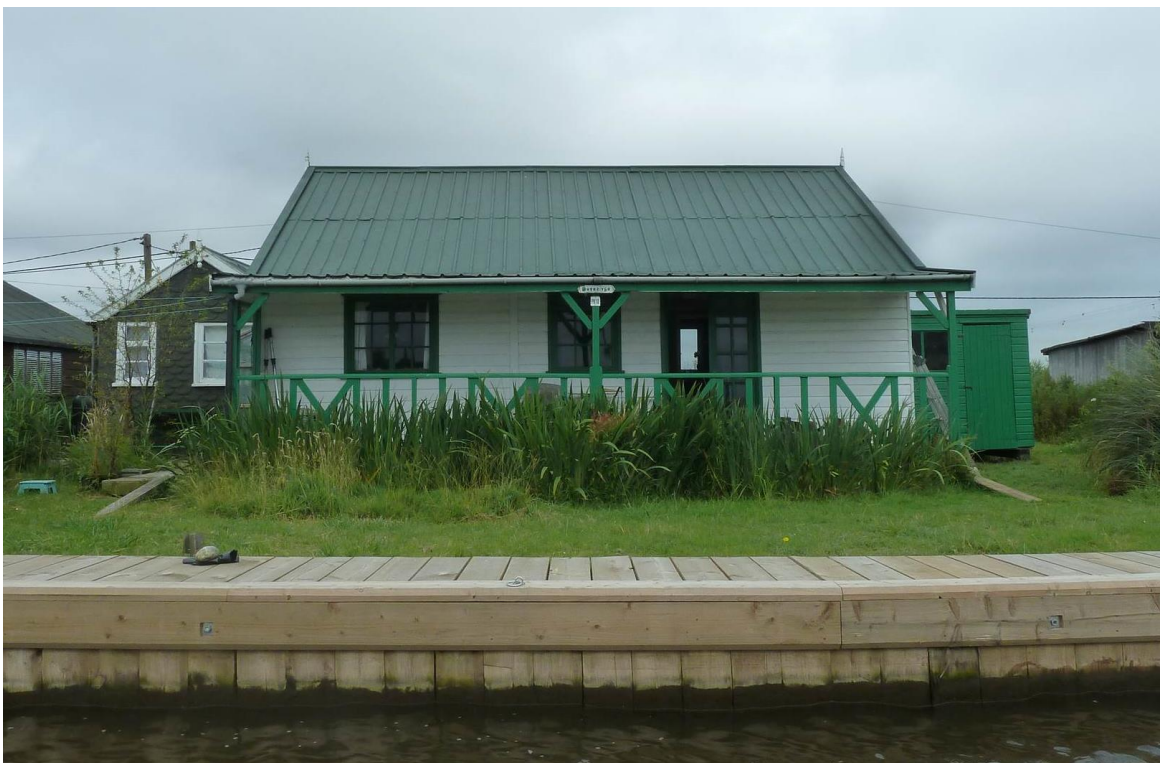
Above: A simple shed-type chalet positioned parallel to the river Thurne at Potter Heigham. The metal roof overhangs a verandah and the building has simple fenestration in a contrasting colour to the timber cladding. There is a decorative timber balustrade and finials on the roof.
