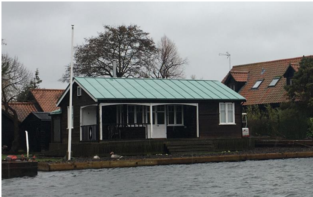
Above: Typical shed-like chalet on the river Bure at Horning. The building has a simple form and fenestration which is painted to contrast with the timber-clad walls, with a profiled metal roof and verandah.
