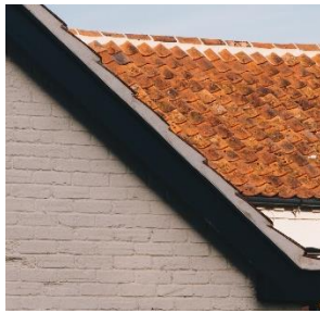
Painted brick, pantiles
