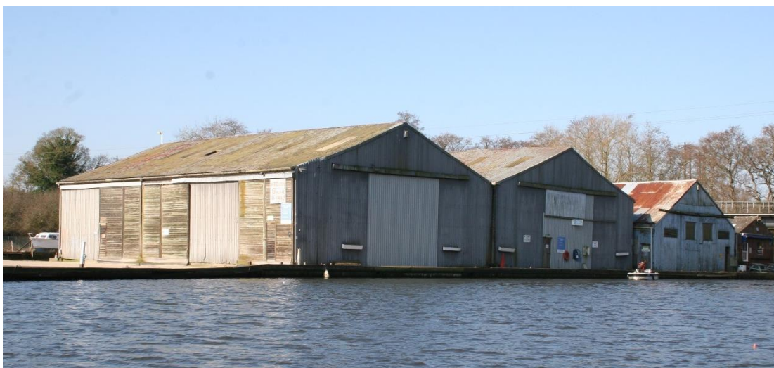
Above: typical boatyards, with large boatsheds of varying heights but similar forms with a prominent gable fronting the water's edge, with the use of metal and timber cladding.
