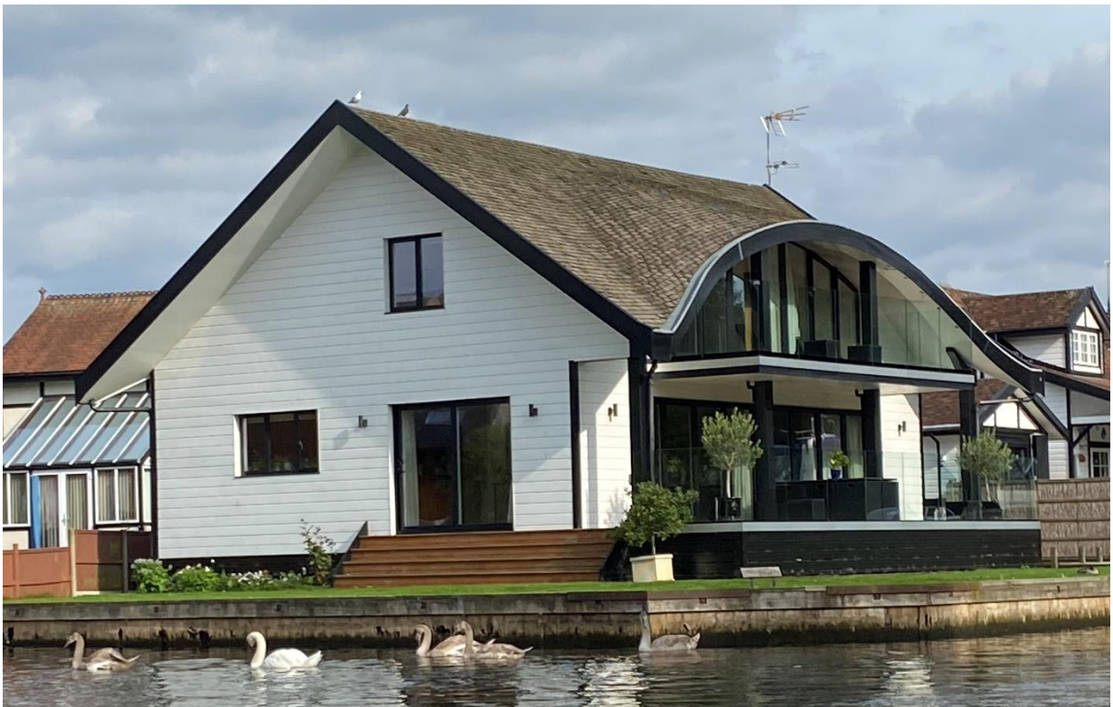
Above: Bide-a-Wee, Hoveton on the river Bure. A contemporary replacement chalet that makes use of traditional materials (timber cladding, shingle roofing) and references traditional details such as the deeply overhanging eaves and an over-sized eyebrow-dormer.
