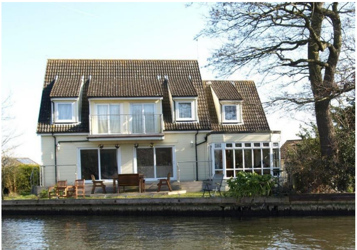
Above: A late 20 th century chalet building of 1.5 storeys, with a steeply pitched roof containing accommodation, lit by dormers. The roof has concrete pantiles and the walls have a light-coloured render.
