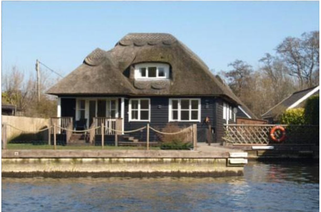
Above: A more recent chalet on the River Bure at Hoveton, also displaying characteristics such as a thatched roof, eyebrow dormer, verandah and simple timber casement windows painted in a contrasting colour to the walls.
