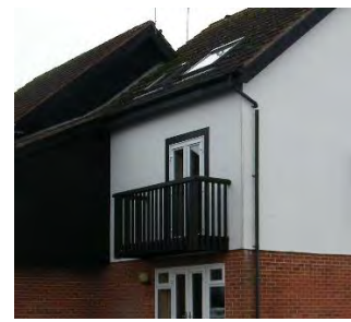
Mix of cladding materials
