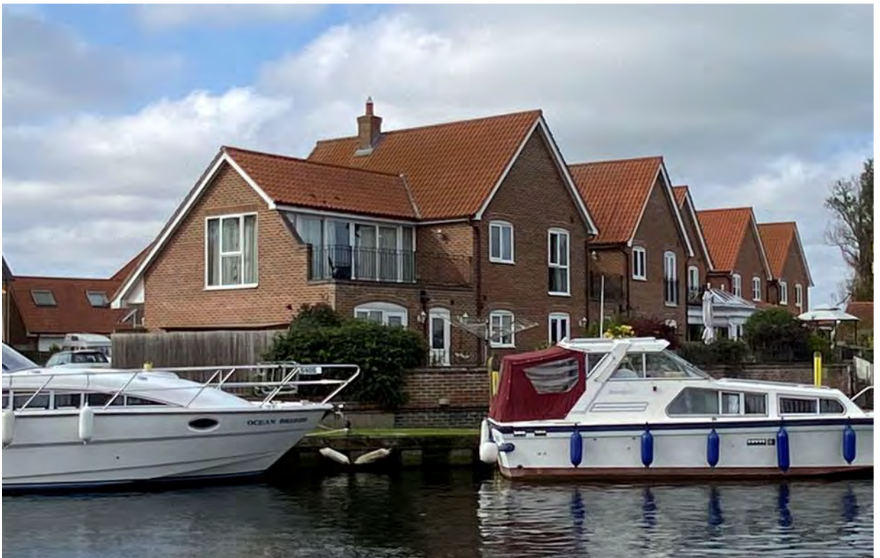
Above: Terrace of waterside (marina) homes in Beccles with typical red brick and varied roof forms, along with a consistency of design.
