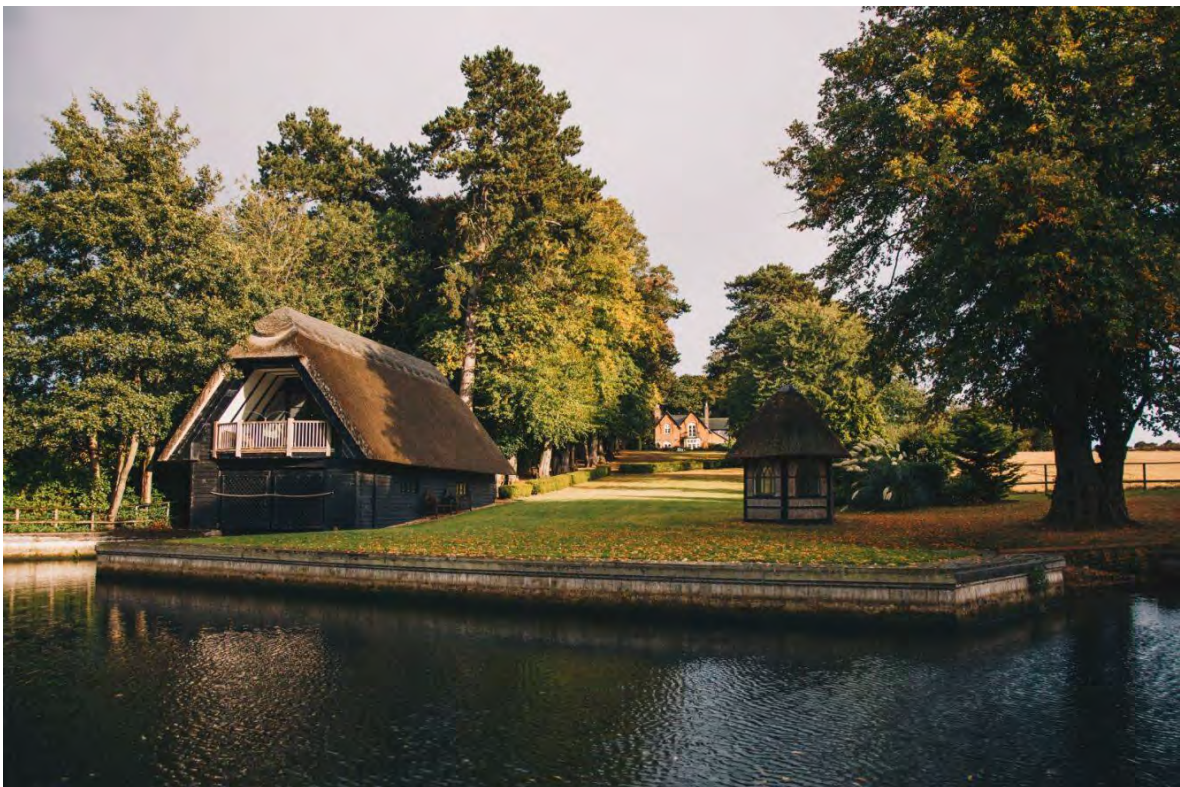
Above: Boathouse, with typical characteristics including use of vernacular materials, low overhanging eaves and inset balcony.
