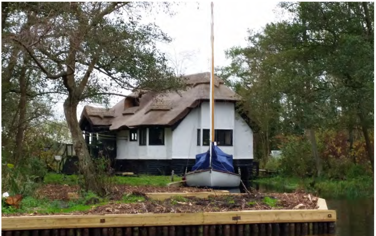
Above: Staithecote on the River Bure at Hoveton demonstrates a number of typical characteristics of the cottage-style chalet, with a thatched roof, deeply over-hanging eaves, timber windows and in this case pargetting.
