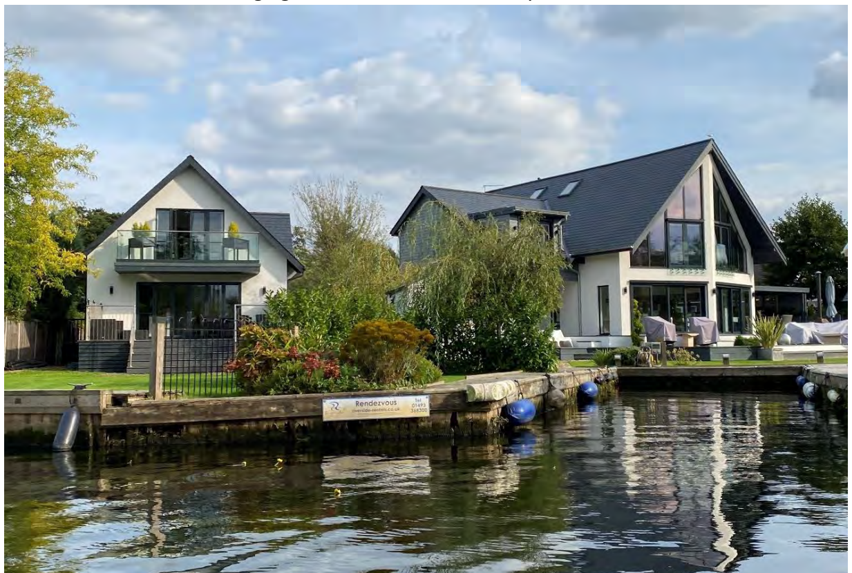
Above: Contemporary chalet buildings on the river Bure at Hoveton.
