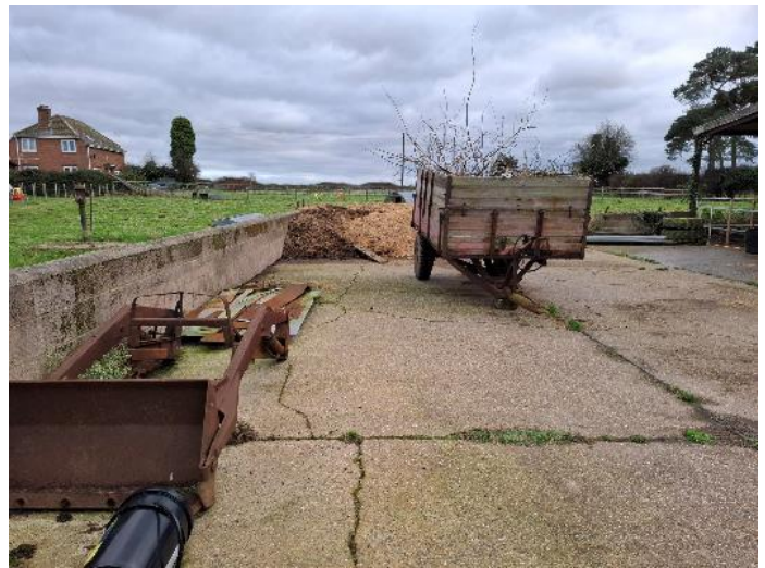
Showing the hard standing and field.
