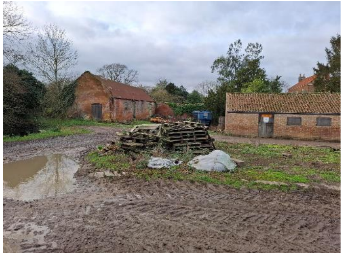
Looking towards farm buildings to the west.
