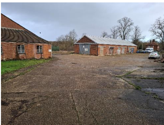
Showing both buildings on site.
