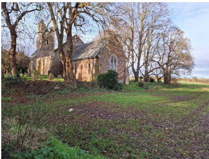
Church on the west boundary of the site.
