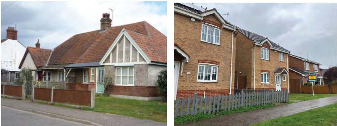
Figure 16- Examples within CA1 from AECOM, 2023
