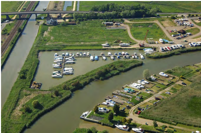
Photo: St Olaves Marina
