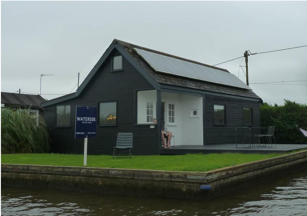
Above: A more contemporary remodelling of a shed-type chalet at Potter Heigham along the river Thurne, where there are predominantly shed-type chalets. This chalet retains the traditional simple form, with timber ship-lap cladding and a verandah.
