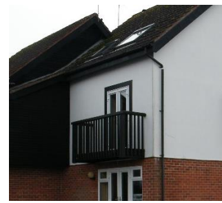
Mix of cladding materials
