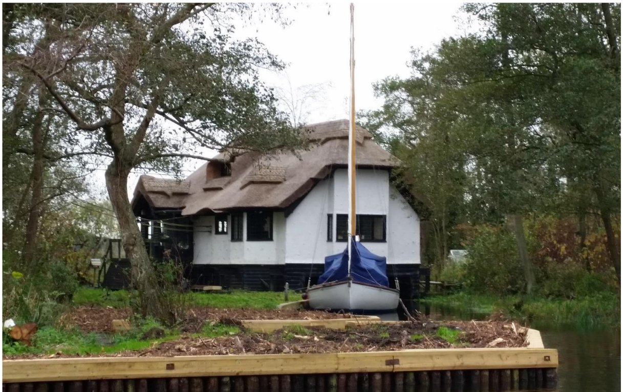
Above: Staithecote on the River Bure at Hoveton demonstrates a number of typical characteristics of the cottage-style chalet, with a thatched roof, deeply over-hanging eaves, timber windows and in this case pargetting.
