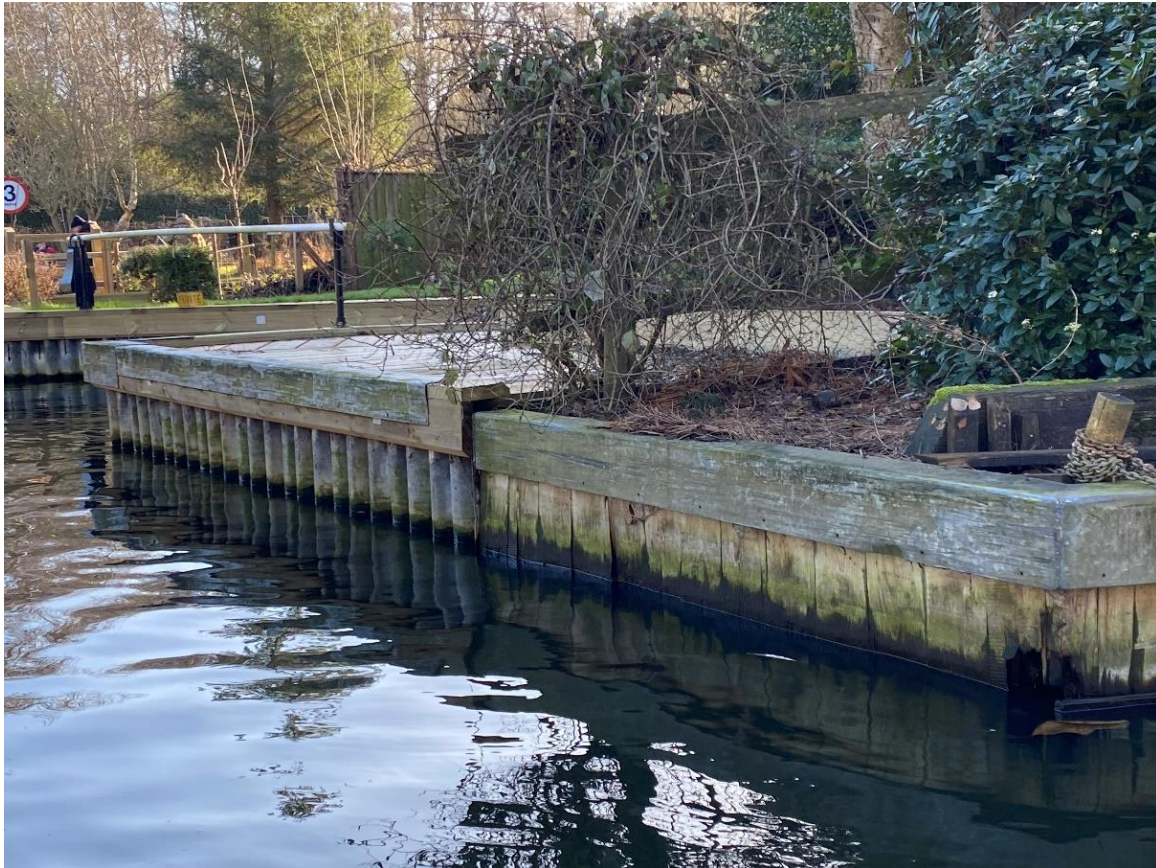
Above: Steel (left hand side) and timber (right hand side) quay heading, both with timber whaling boards and capping.
