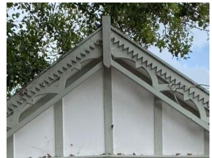
Timber-framing and render
