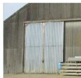
Metal sheet cladding
