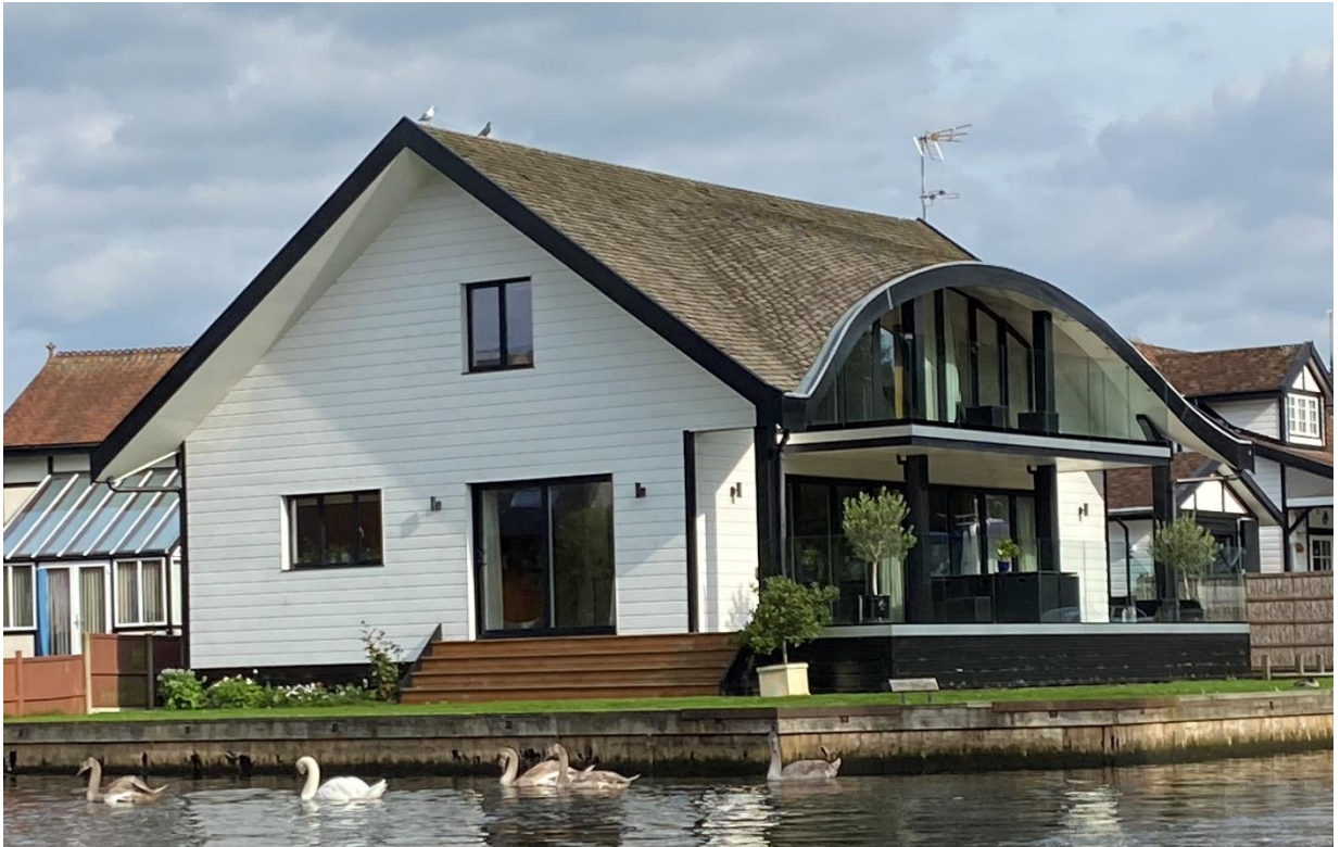
Above: Bide-a-Wee, Hoveton. A contemporary replacement chalet that makeuse of traditional materials (timber cladding, shingle roofing) and references traditional details such as the deeply overhanging eaves and an over-sized eyebrow-dormer.
