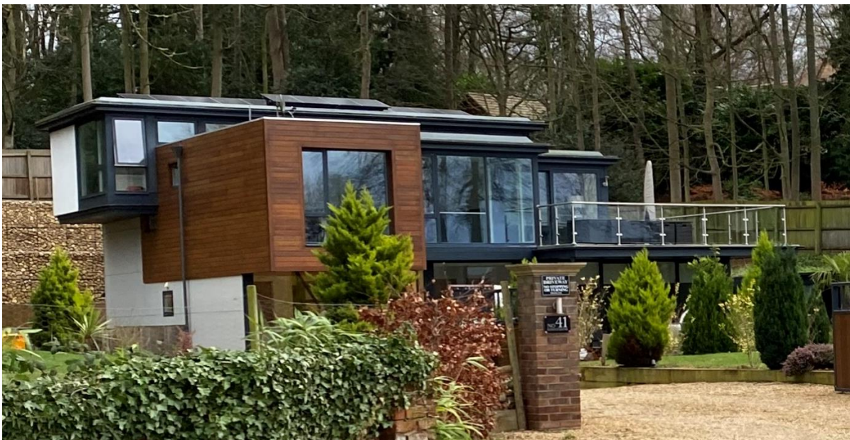
Above: Flat roofs can on occasions be considered appropriate for contemporary waterside homes
