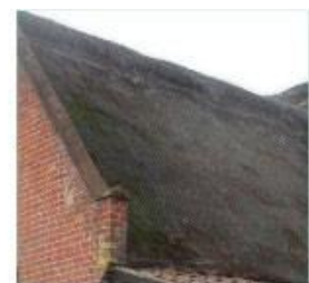
Thatch and parapeted gables
