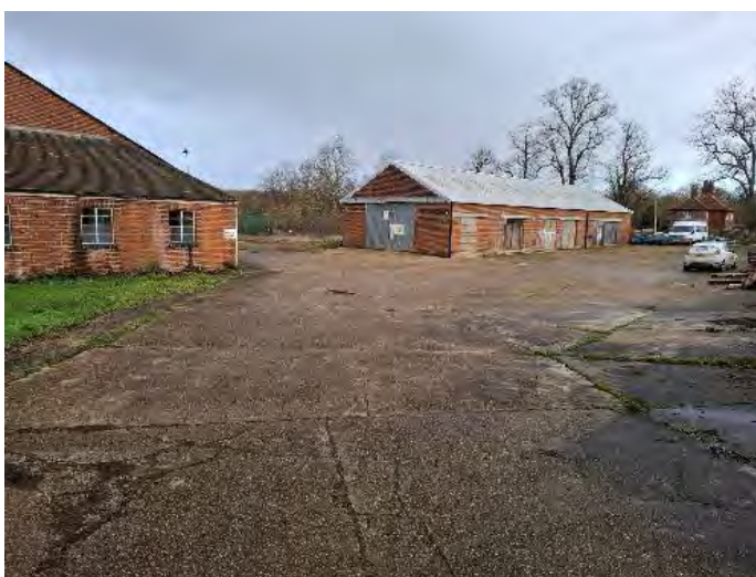
Showing both buildings on site.
