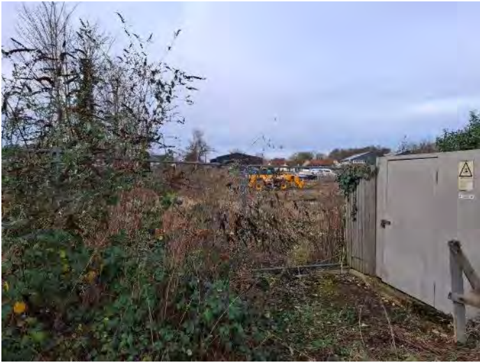
Utilities infrastructure on the right
