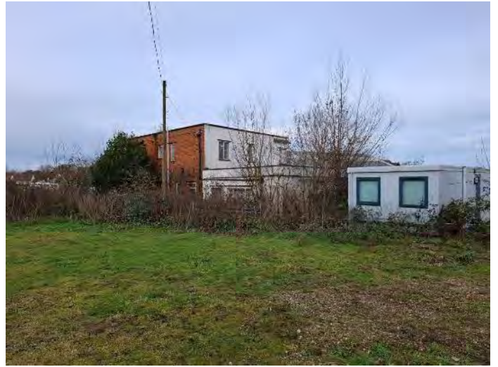
Looking north at the buildings on the site
