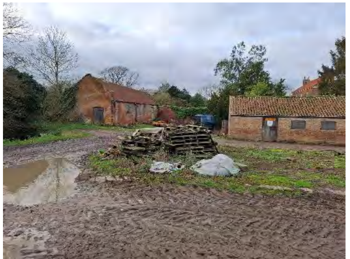
Looking towards farm buildings to the west.
