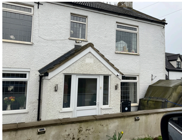
Figure 44: The use of uPVC windows should be avoided, regardless of their design.
