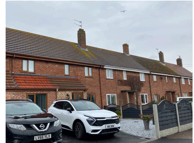
Figure 23: Terraced housing on Church Road.
