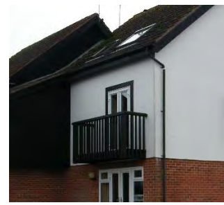
Mix of cladding materials
