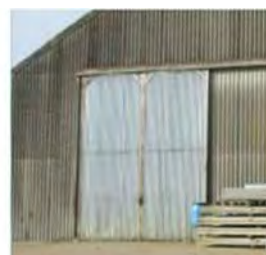
Metal sheet cladding
