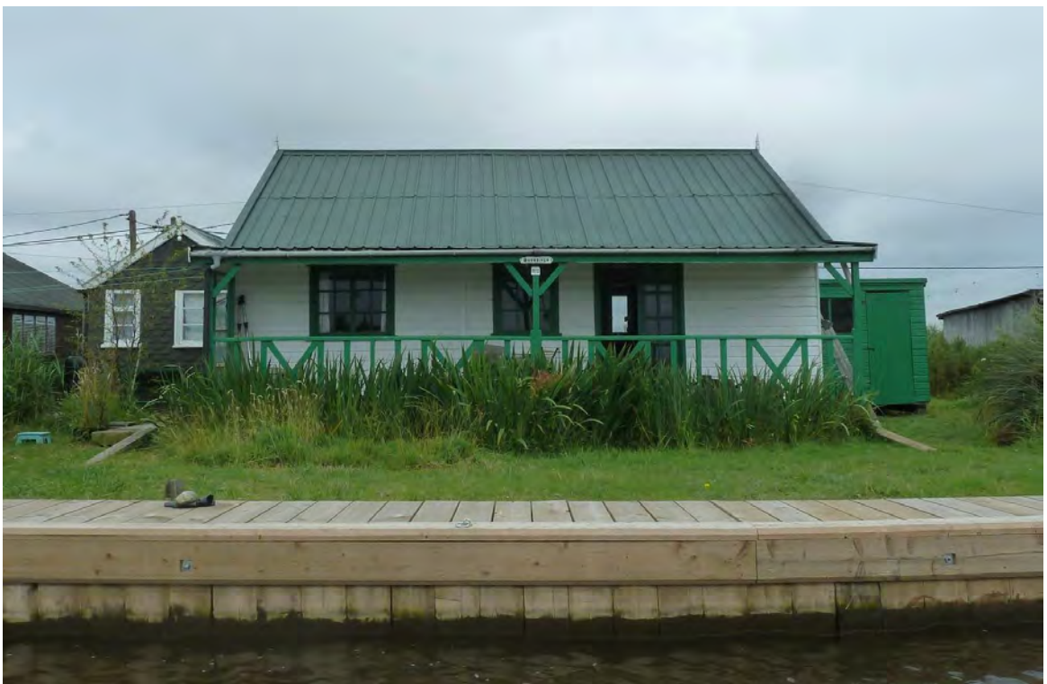
Above: A simple shed-type chalet positioned parallel to the river Thurne at Potter Heigham. The metal roof overhangs a verandah and the building has simple fenestration in a contrasting colour to the timber cladding. There is a decorative timber balustrade and finials on the roof.
