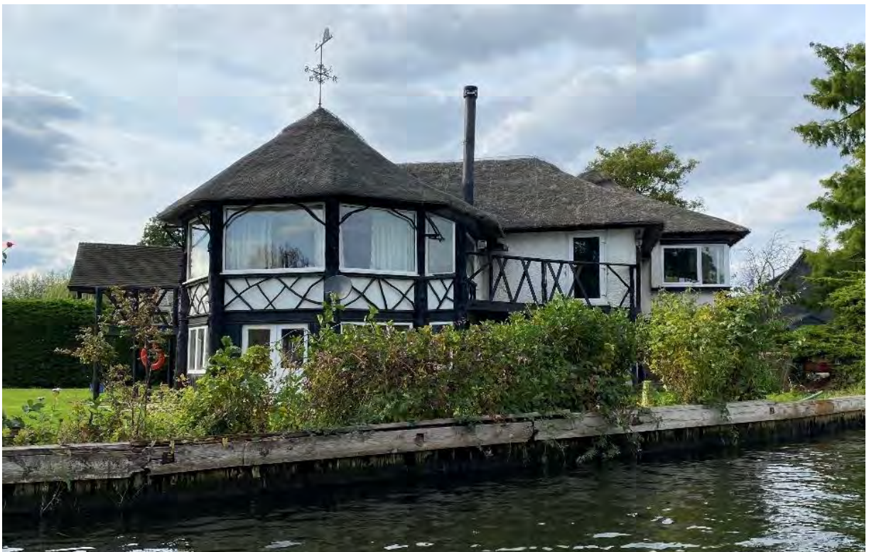
Above: The Beehive at Hoveton is a slightly larger two storey cottage-style chalet that also has a thatched roof, render with applied timber framing and rustic un-hewn timber framing.
