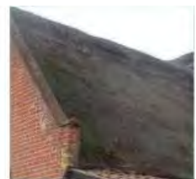
Thatch and parapeted gables
