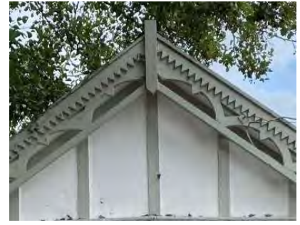
Timber-framing and render
